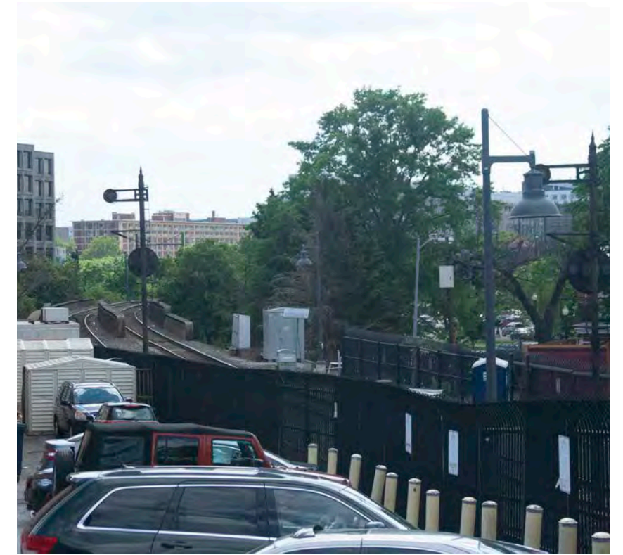
view southwest along railroad tracks
