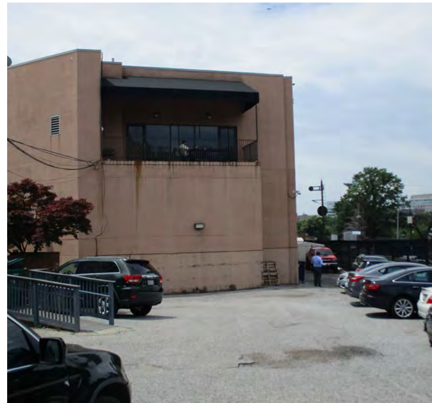
structure in alley to southwest
